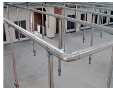
Drops to the point of use, are fast and easy to assemble or modify.
