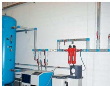
Aluminum distribution pipe for compressed air, vacuum and other non dangerous gases, from 20 to 110 mm diameter.
